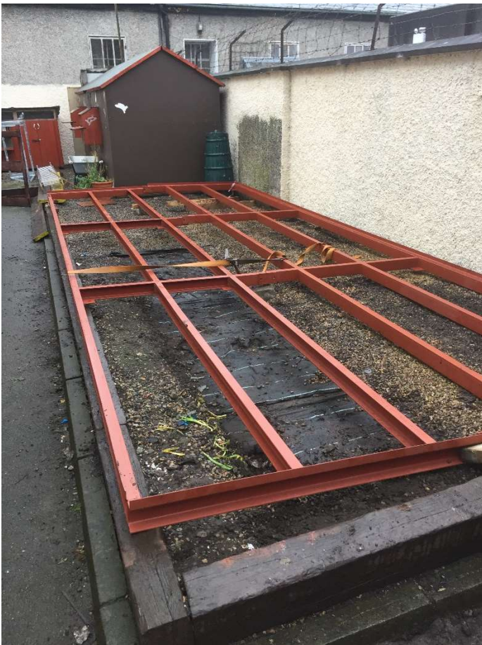
Base Frame installed and levelled.
