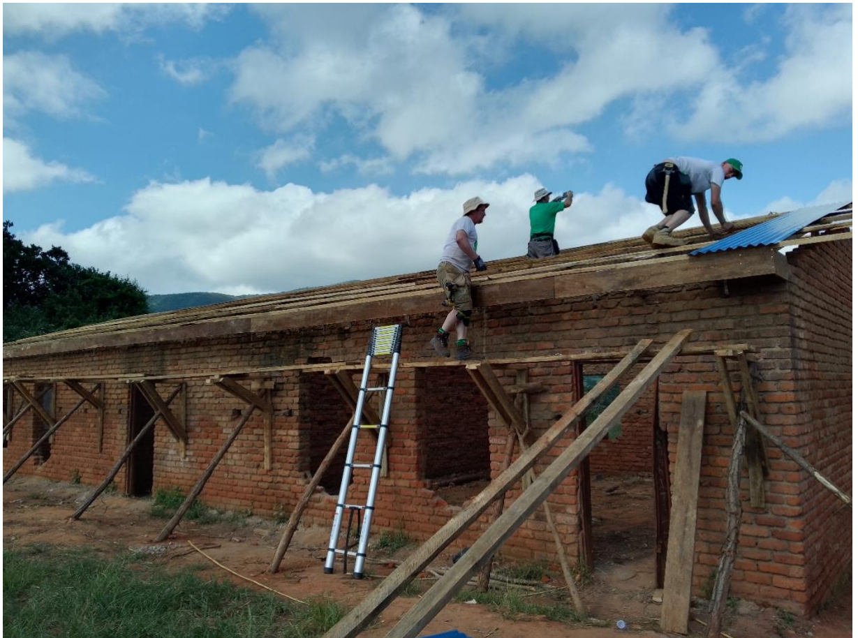
Timber works completed and starting sheeting works
