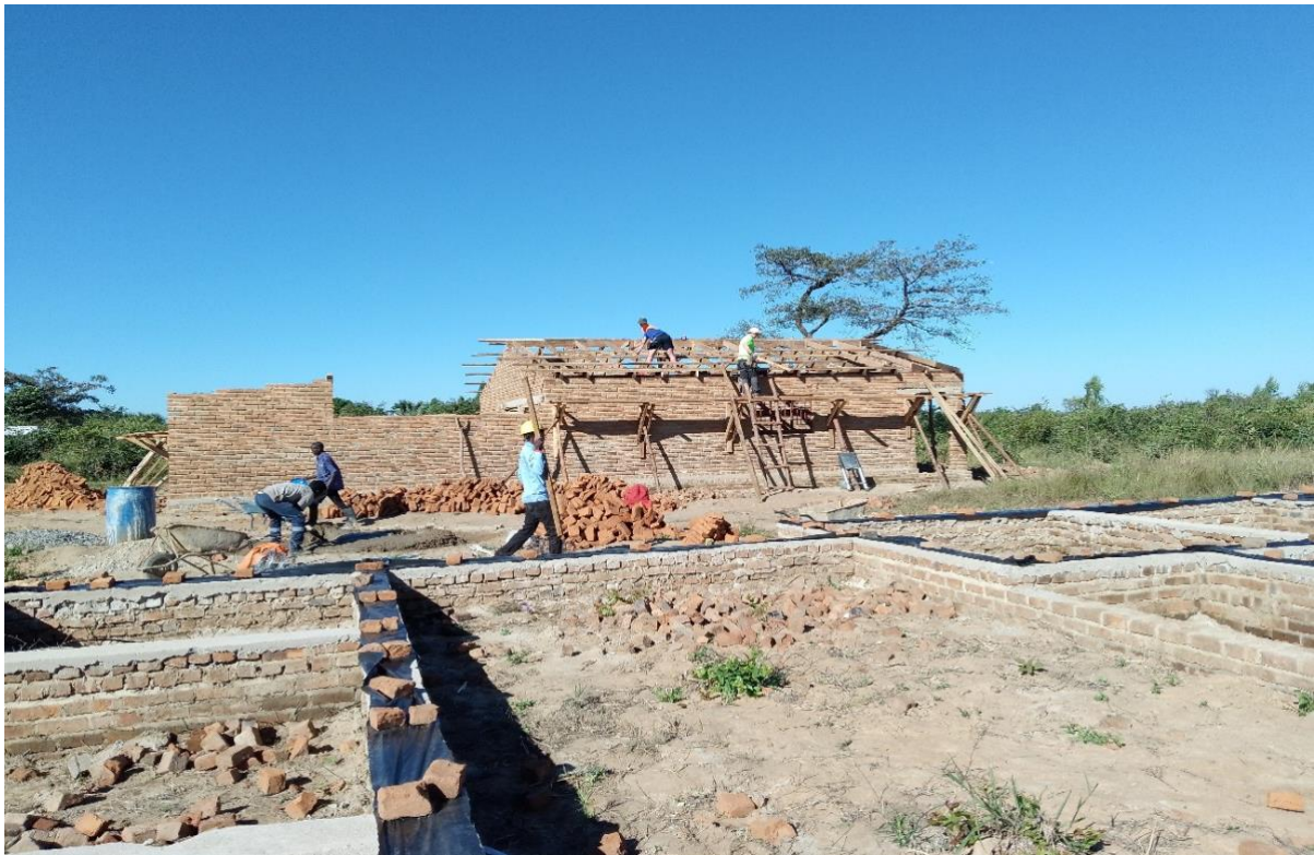
Kameva Teachers' house timber work
