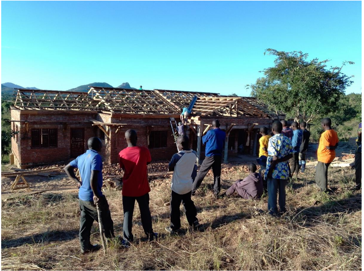
Timber works completed
