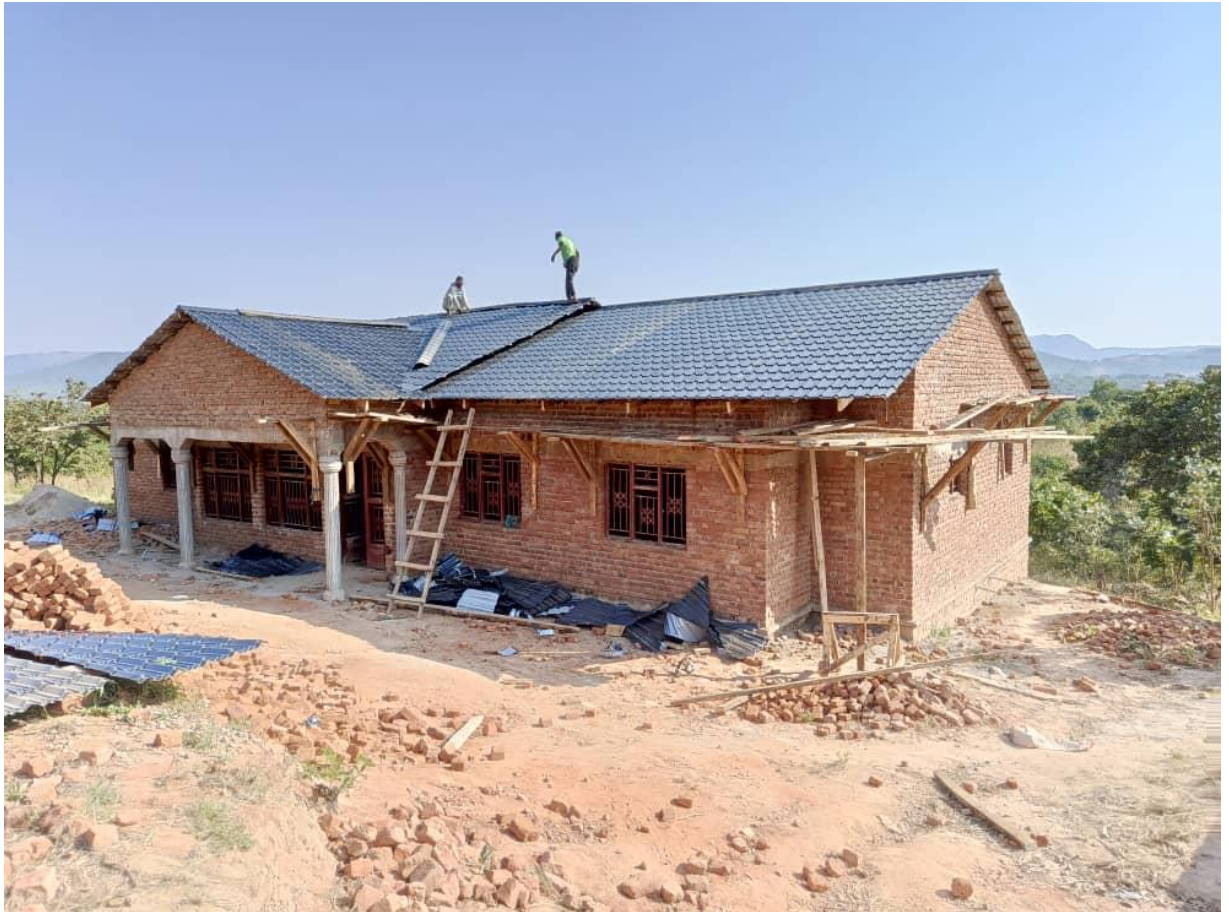
Completion of sheeting by local carpenters.
