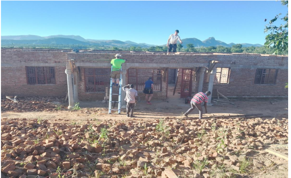
Setting up the roofing works – Father’s house – Chizani
