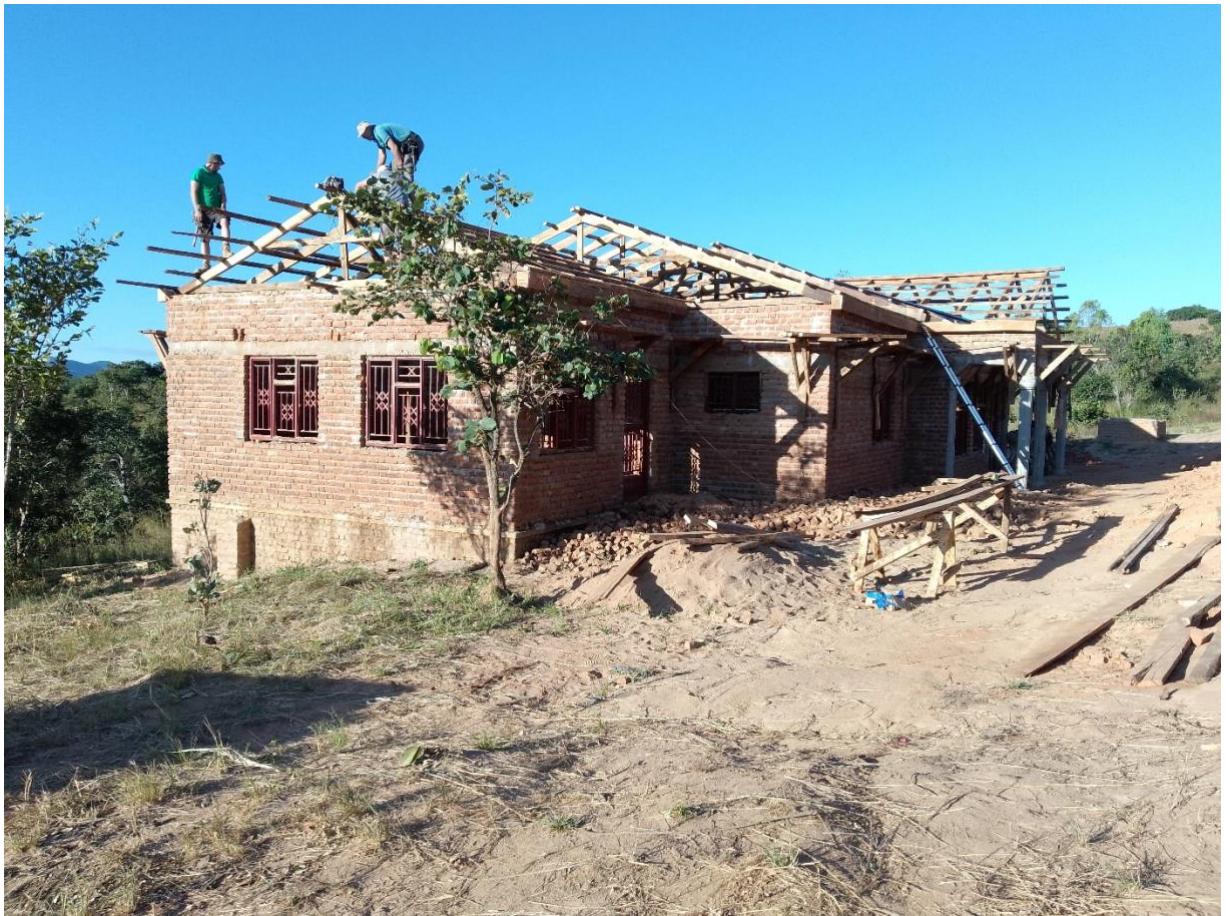
Timber works in progress – Father’s house
