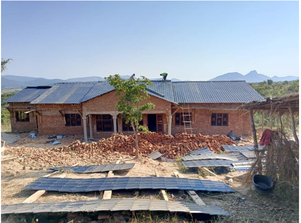
Front view – completing of sheeting by local carpenters.
