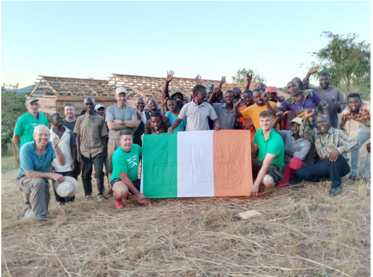
Celebrating completion of timber works at Chizani – Father’s house
