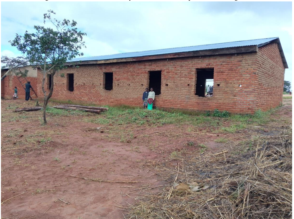
Back view of the roofed classroom block
