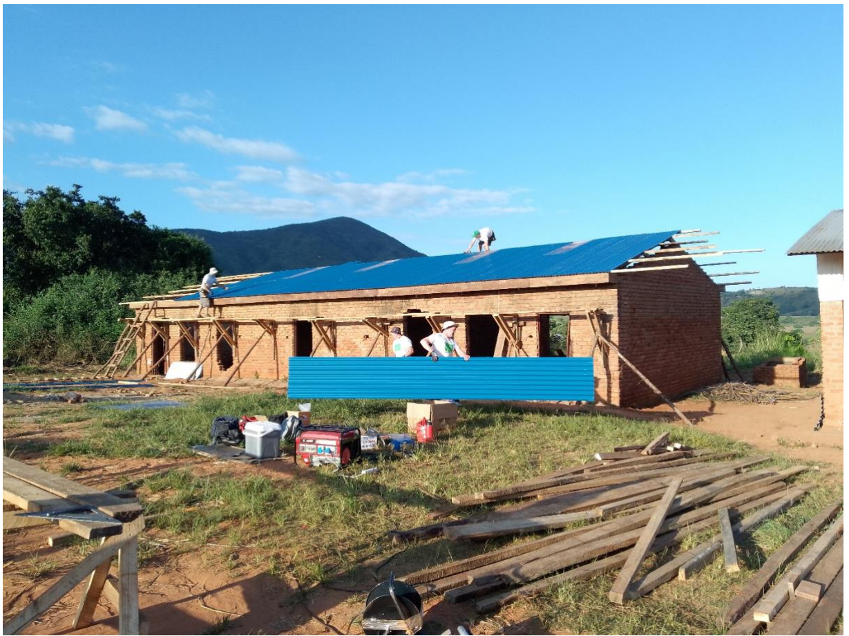
Sheeting works in progress
