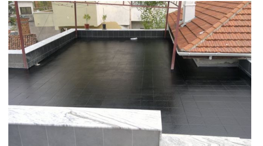
Convent roof in Tirana receives bitumen sealer
