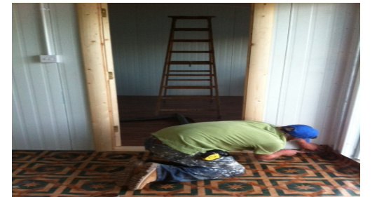
Skirting, architrave and lino fitted to all houses
