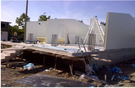
Construction begins on this new house
