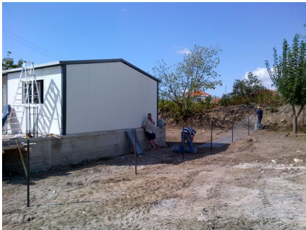
Perimeter fence installed around the house.
