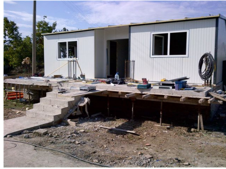
Windows and doors installed
