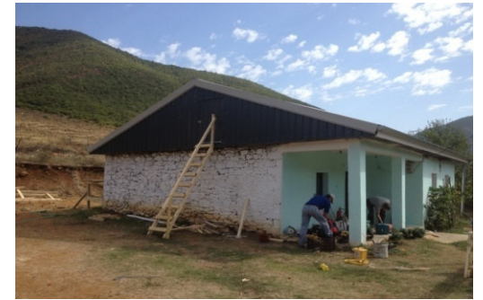
Roof completed and access ladder to attic area fitted.
